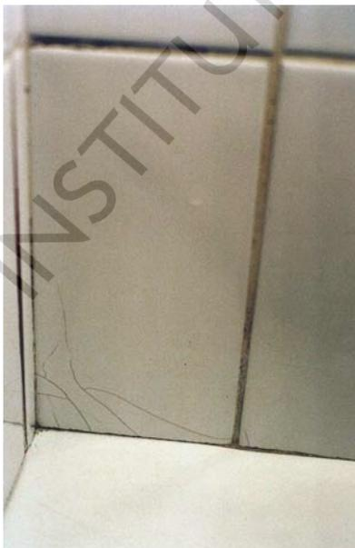
*Crazing in BIII GL tile, at the juncture with the sanitary ware and change of plane*
